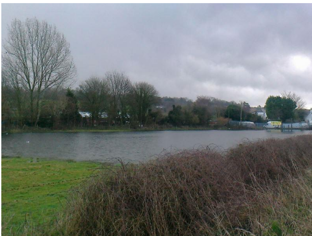
Photograph 7: Groundwater emergence & extensive ponding
