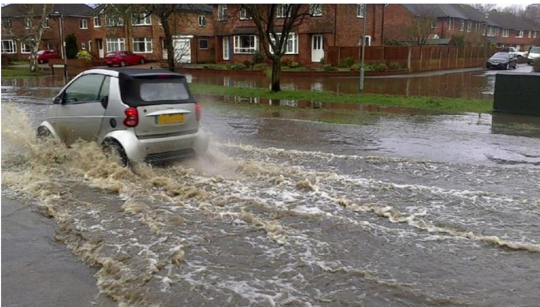
Photograph 1: Floodwater affecting the highway
