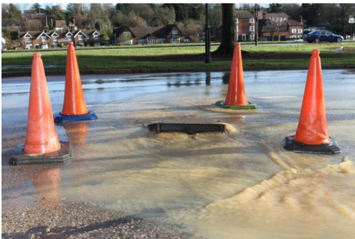
Photograph 8: A surcharged manhole (the sewer system has reached its capacity and water now escapes via manholes)
