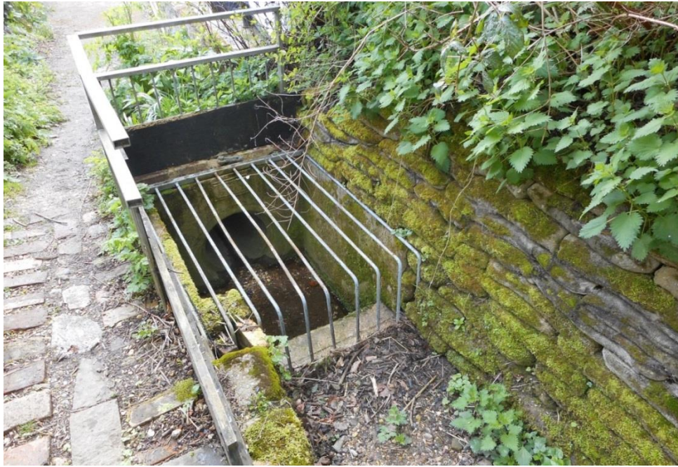
Photograph 6: A culvert on a small watercourse
